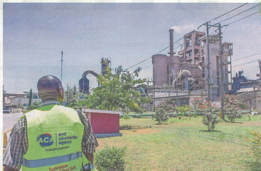
Bamburi Cement factory in Mombasa. The firm's turnover for 2021 went up 19 percent to $414 million from $349 million the previous year.
