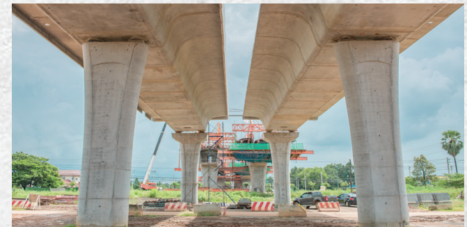
Deep rafts, Windmill foundations, Large Beams, Columns & Slip Form Works
