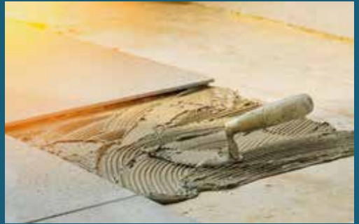
Internal tiling on floors
