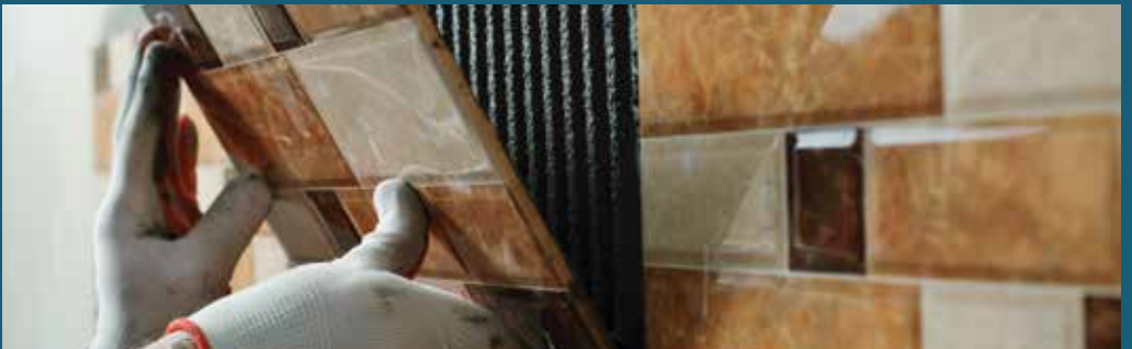
Tile repairs and rehabilitation works
