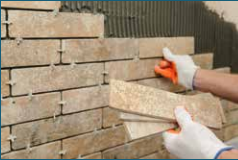
Internal tiling on walls
