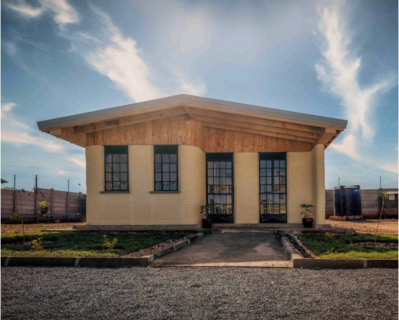
Bamburi Cement in partnership with 14 Trees launched the 1st 3D Printed house in Kenya last year
