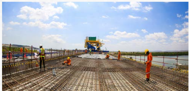
Dongo Kundu Bypass in Mombasa
